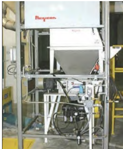
Stainless steel batching station for both bulk bags and drums
