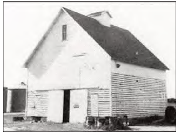
The warehouse was in the corn crib alley
